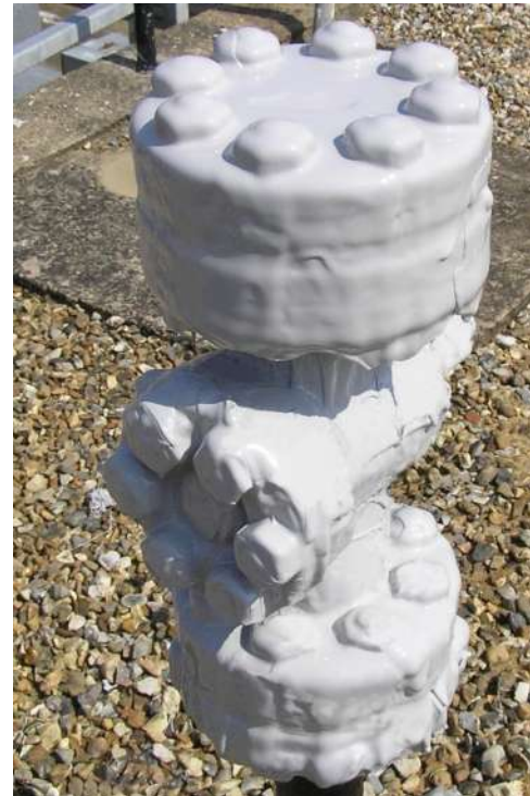
Multiple flanges encapsulated using ENVIROPEEL
